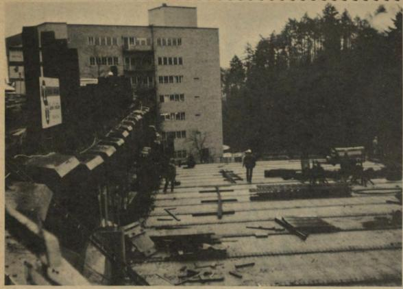
▲ Temporarily slowed down by bad weather, construction on the new 787-space parking structure has resumed. About 10 per cent of the 320 lintees (pre-cast flooring) have been laid, over which will be poured three to five inches of cement formed for drainage.
