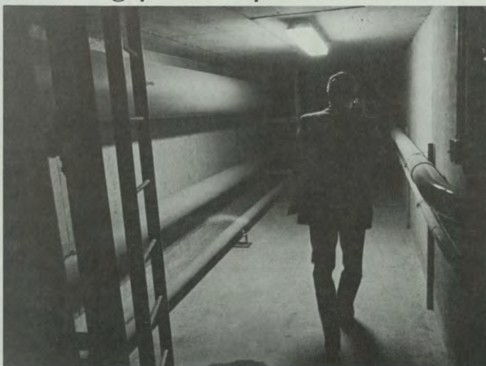
A labyrinthine tunnel system will one day connect all areas of the Health Sciences Center. The first tunnel, connecting the new heating plant with a point near Veterans Road, has been completed in conjunction with construction of the new plant.
