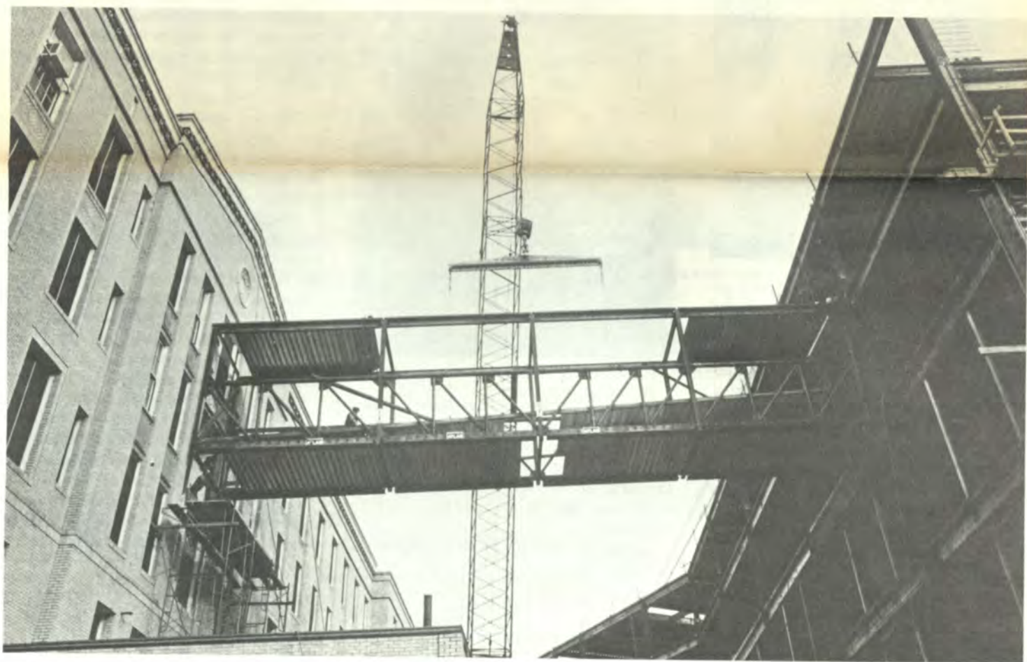
Workers connected University Hospital (north) with the new Shriners hospital in February by raising a 23-ton sky bridge into place. The 70-foot
