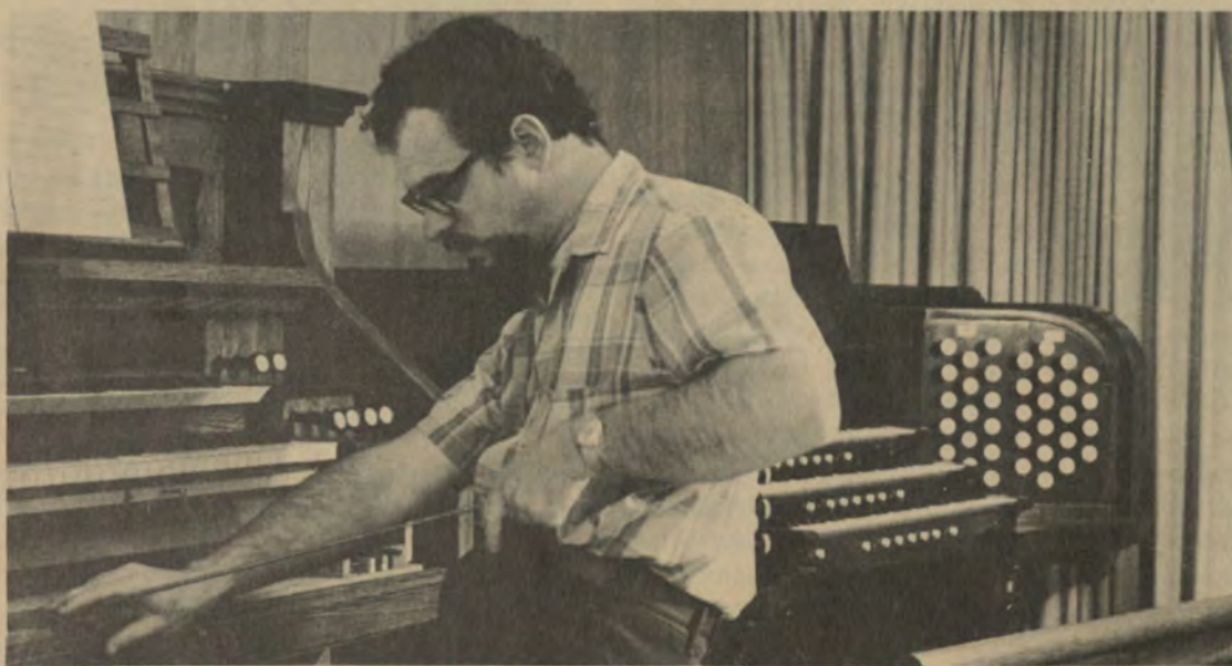
Seated at the console of his reed organ, Bud Wilkinson has removed a panel under the keyboards and is using a "reed puller" to extract a reed for cleaning; there are more than 500 reeds in this organ.
