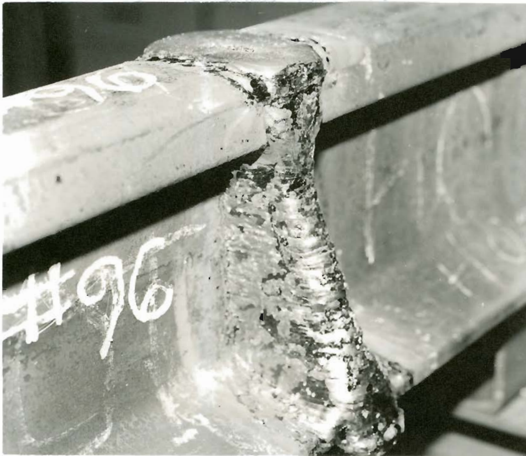
Figure 17. ELECTROSLAG RAIL WELDING SETUP AND COMPLETED WELD.
